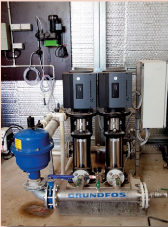
The irrigation system includes two Grundfos multi-stage pumps with Hunter ACC controller
