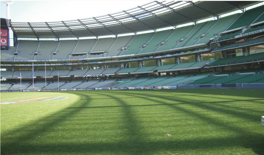
Despite its transparent roof, the new stand will have major implications for the MCG surface, particularly in regards to shade management
