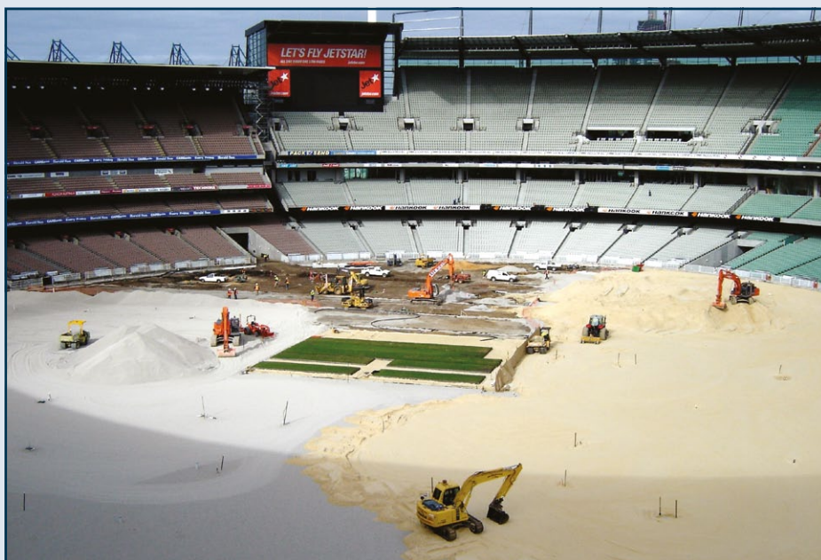
Placing the gravel drainage blanket and rootzone sand
