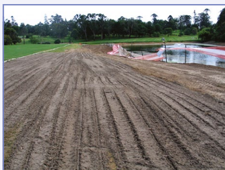
Work on the 18th fairway at Castle Hill
