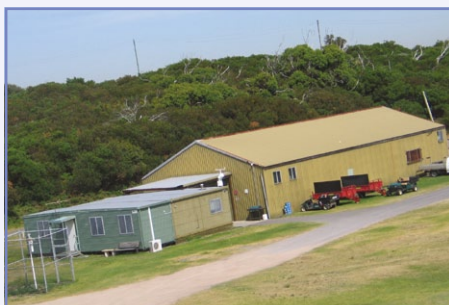
The soon-to-be-demolished "temporary" NSW maintenance facility
