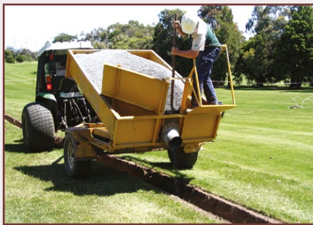
A modified tipper trailer has made drainage issues a thing of the past at Ringwood Golf Course
