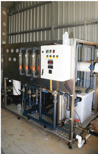
Wesley's desalination unit produces 48,000 litres a day at 250ppm
