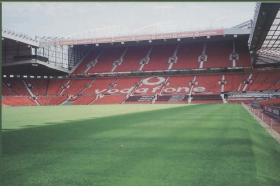
The translucent stadium roof at Old Trafford allows partial light to filter through to the turf, helping reduce the impact of shade
