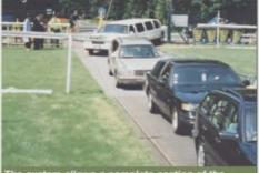
The system allows a complete section of the racetrack to be moved to reveal the road beneath enabling traffic to pass without damaging turf.
