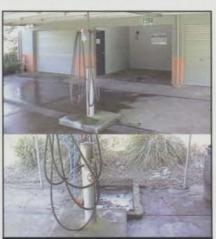
A new washdown facility installed at the Lakelands Golf Club in Queensland collects rinsate from chemical application and other maintenance equipment separately and separators are used to take out oils and solids. Rinsate from the chemical storage area and the chemical washdown pad is passed through to an 8000 litre holding tank. A 2000 litre spray tank siphons contaminated water from the holding tank and using a handgun, the water is sprayed out along the fence lines.
