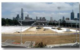
A flat cell drainage system was designed to avoid trenching into the contaminated subgrade
