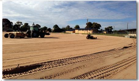
Some 9700 tonnes of rootzone sand was imported to the site and amendments power harrowed to a depth of 100mm. The surface was then rolled and given a final trim
