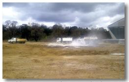
A decision was made to incorporate lime into the profile to help stabilise the subgrade and stiffen up any soft spots
