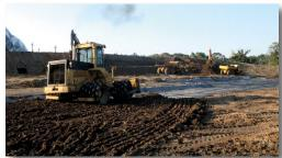
A large sheepsfoot roller was used to compact the subgrade layers and remove any voids
