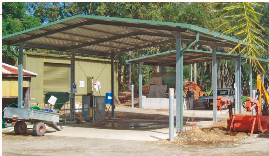
Covering the wash bay with a roof eliminates rain ingress
