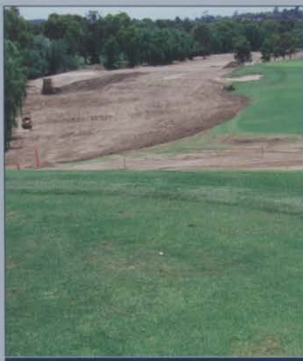
Construction of the new 1st at Freeway
