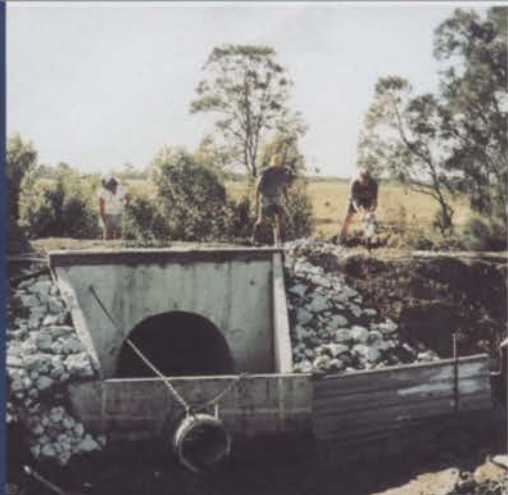
Groundstaff constructing weir
