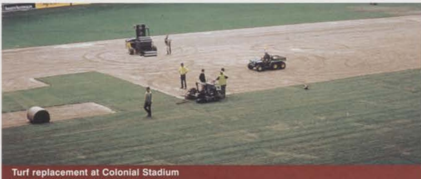
Turf replacement at Colonial Stadium
