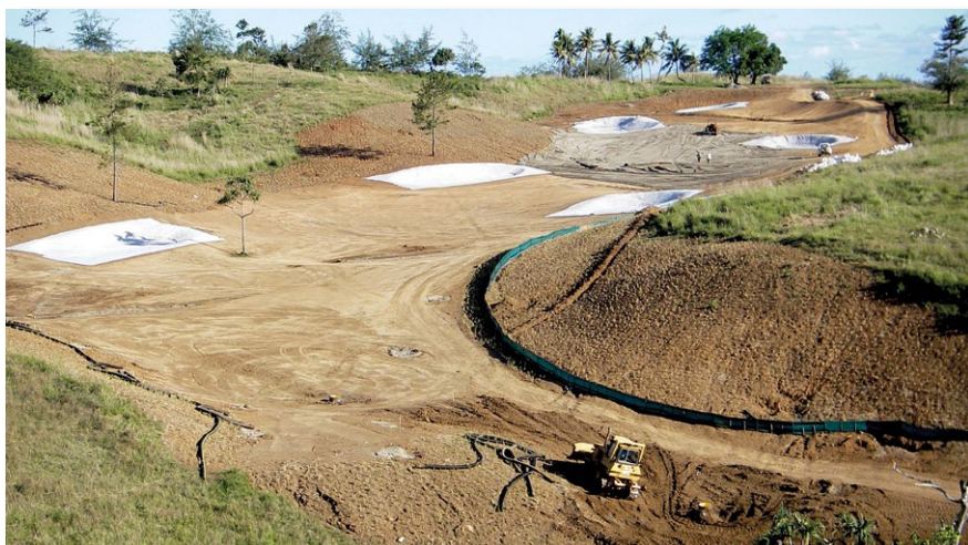
Natadola was built to USGA specifications with the fairways sandcapped at a depth of 300mm due to the underlying limestone rock
