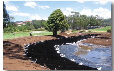
Construction of the lined irrigation pond which stores treated effluent
