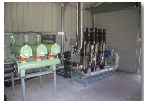
Byron Bay Golf Club installed a variable speed Rain Bird V-3300 pump which increased capacity to 30l/s
