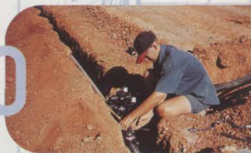
← HUNTER 31 SPRINKLER HEADS AND TORO OASIS PTC 42 CONTROLLERS BEING INSTALLED
