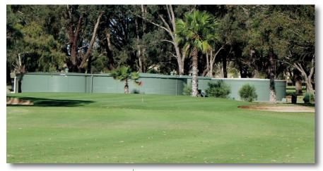
A series of eight water tanks are used to store a mix of effluent water from the local treatment plant and bore water
