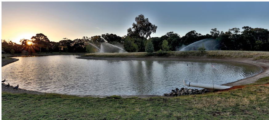
Deniliquin's new 22ML holding dam which stores both river water (from Edward River) and stormwater run-off from the township
