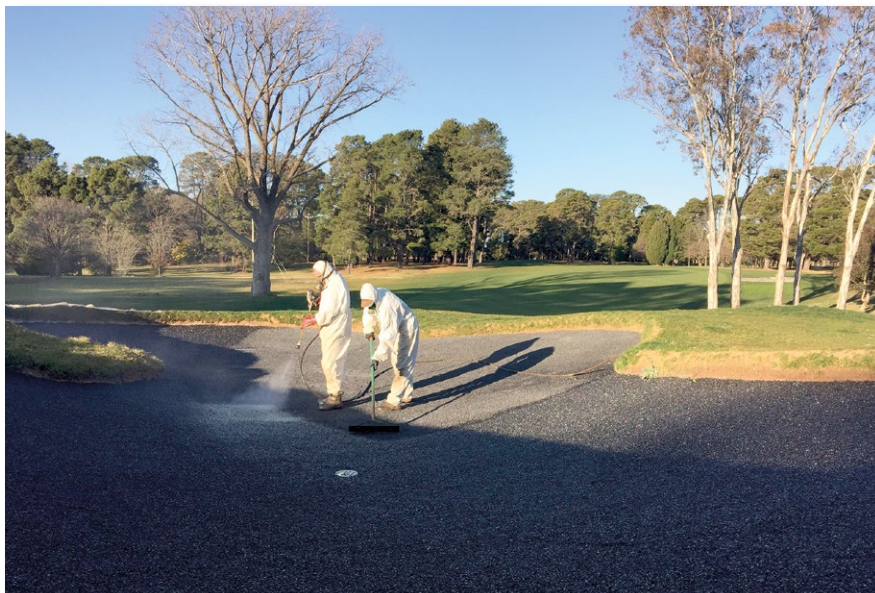
The new Royal Canberra bunkers have had Kustom Bind installed
