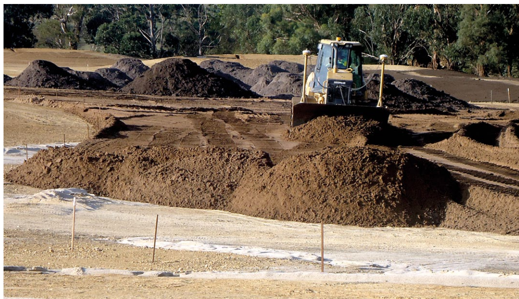
A dozer fitted with GPS receivers on the blade pushes out fairway sand over the shaped subbase on the 2nd fairway. Around 27,500m 3 of imported sand has been used to cap fairways
