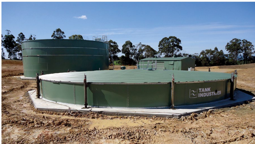
Construction of the onsite 1ML storage tanks showing the hydraulic lifting mechanism used to raise the tank up as further layers are added. The course will be irrigated with Class B recycled water from the adjoining Lilydale treatment plant
