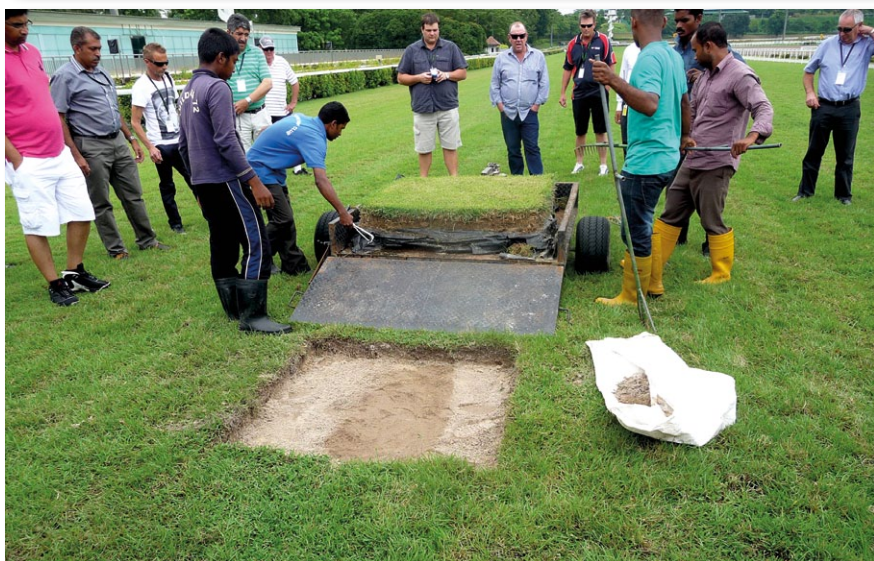
Top: The 15cm wide x 10cm deep Reflex reinforced plug used at Singapore's Kranji racetrack. Grown in steel rings, its straight sides and 100mm depth means that even with immediate racing the new plug is not displaced
