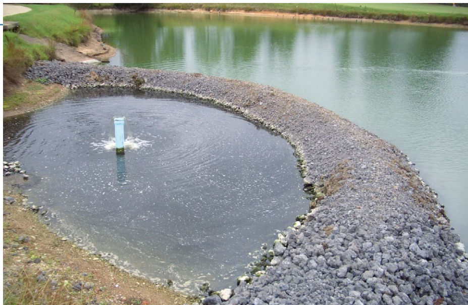
The installation of a permeable reactive barrier combined with the rafted reedbeds has seen a dramatic improvement in water quality at Catalina Country Club
