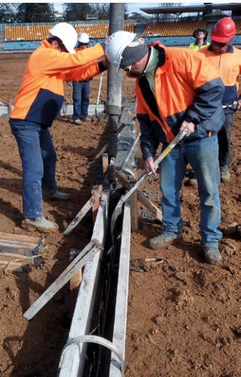
The first stage of the wicket construction saw a concrete retaining wall built to encase the wicket soil and hold it in place. The top of this wall is 150mm below the finish level
