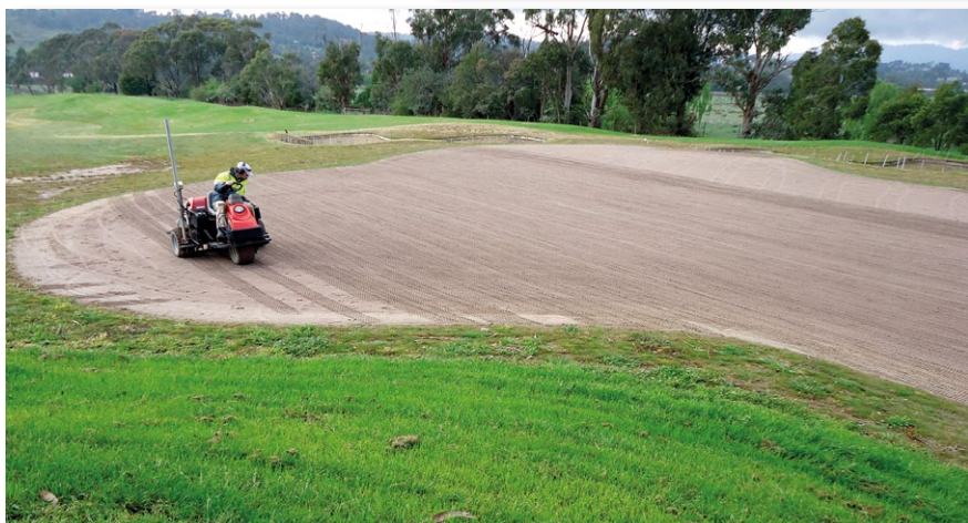
After seeding, greens were tyre rolled with a bunker rake
