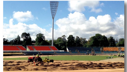
4500m 3 of sand was brought in with the top 140mm amended with 5 per cent cocoa fibre
