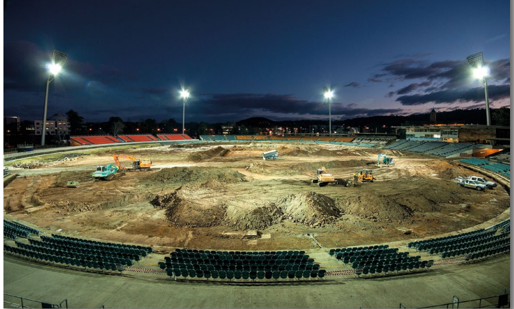
Above: Stage one of the arena upgrade saw the installation of six 47 metre broadcast quality light towers during the 2012/13 summer
