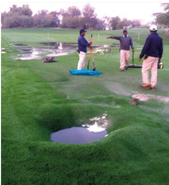
A mainline blowout on the 12th four weeks out from this year's Masters
