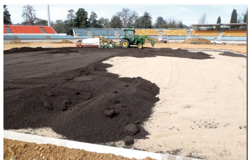
The first stage of the wicket construction saw a concrete retaining wall built to encase the wicket soil and hold it in place. The top of this wall is 150mm below the finish level
