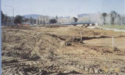
PRECONSTRUCTION DURING EARTHWORKS
