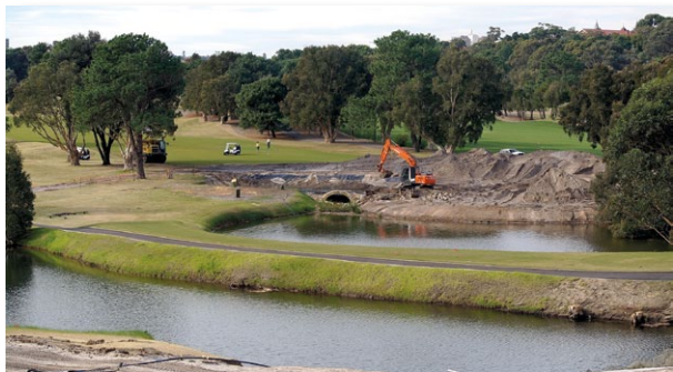
The 7th green during and after reconstruction. The 7th received major reworking, with the green complex dropped by 1.5m to not only provide a better look through the green but also open up the lake on the right hand side. A bail out area was also incorporated to the left of the green
