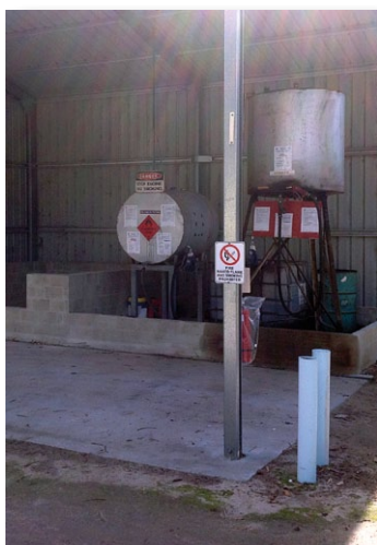
Careful planning and budgeting has enabled Busselton to recently construct a new washdown/chemical mixing area and a specialised banded fuels and oil storage area
