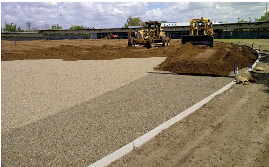
◀ The new design included a 300mm USGA-spec rootzone sand profile
