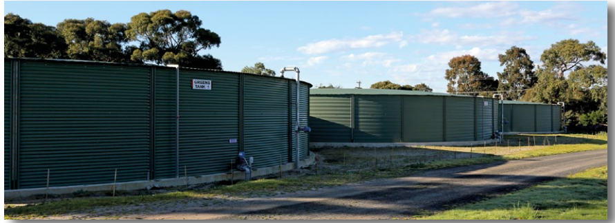
To remedy a lack of water storage capacity, three 1ML tanks were constructed on a property the club owns adjacent to the course. The low profile tanks store the sulphur-treated water used for greens irrigation
