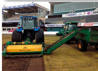
After spraying out the oval with Roundup and milling the outfield to a depth of 50mm (above), treading of the Blundstone Arena surface (below) started on 23 July 2012
