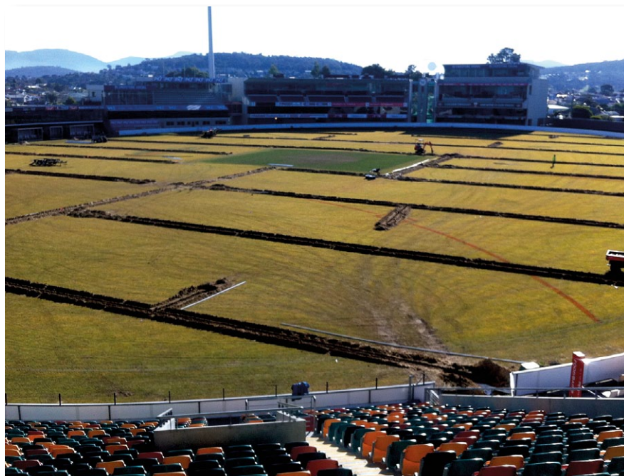
After spraying out the oval with Roundup and milling the outfield to a depth of 50mm (above), treading of the Blundstone Arena surface (below) started on 23 July 2012
