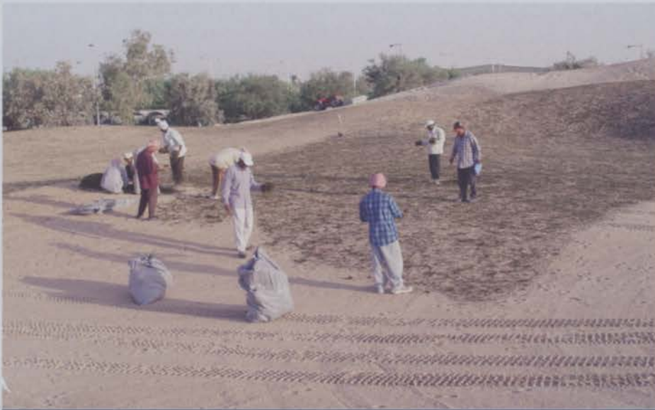
Due to extreme day-time temperatures in Kuwait, most sprigging was carried out late in the day and at night time
