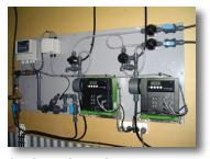
On-site dosing units, such as this one at Cataline Country Club, can be used to buffer pH and displace sodium, along with using surfactants.
