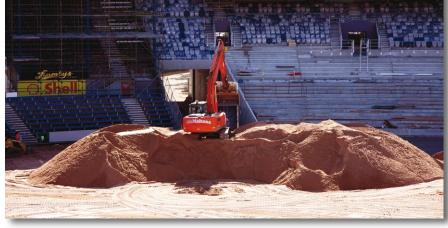
place to do so outside of the ground due to the stand construction. From there a 20 tonne excavator would fill small 'moxy' trucks to take the material around the oval. Considering the moxys only hold 2m³ at a time, it was a Herculean effort.
