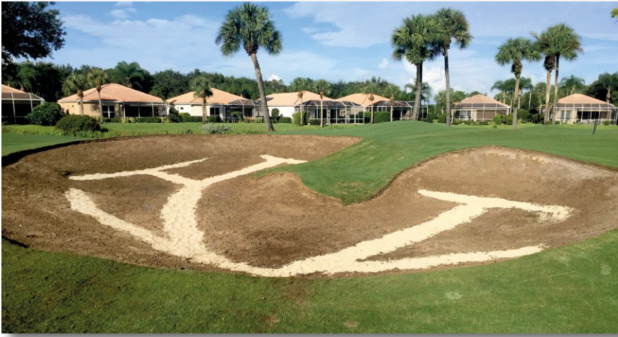
With an annual rainfall of nearly 2m, drainage was a key focus of the Vanderbilt renovation
