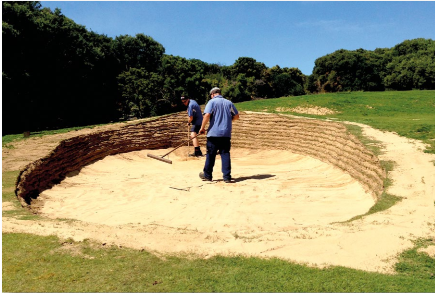
◀ The new revetted bunker on the 10th
