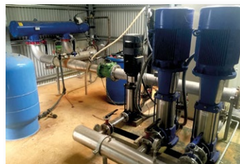
The Toro irrigation system is fed by three Grundfos pumps which can push out 1600 litres per minute at full capacity
