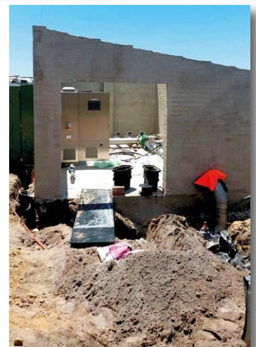
The installation of five new Grundfos submersible pumps and a new pump house formed a major part of the first stage of the project
