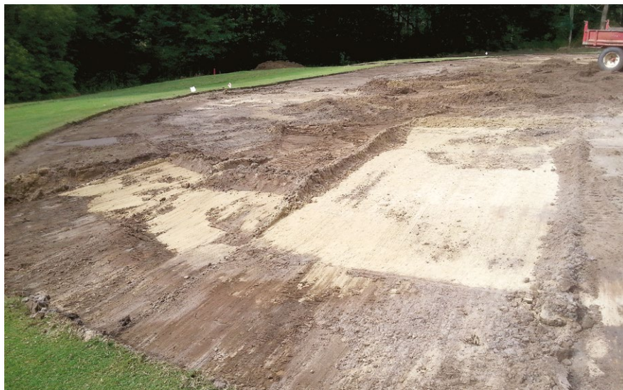
The old 15th green showing layering within the profile that was restricting the performance of some of the greens
