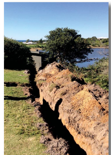
Mainline trench from the pump house
