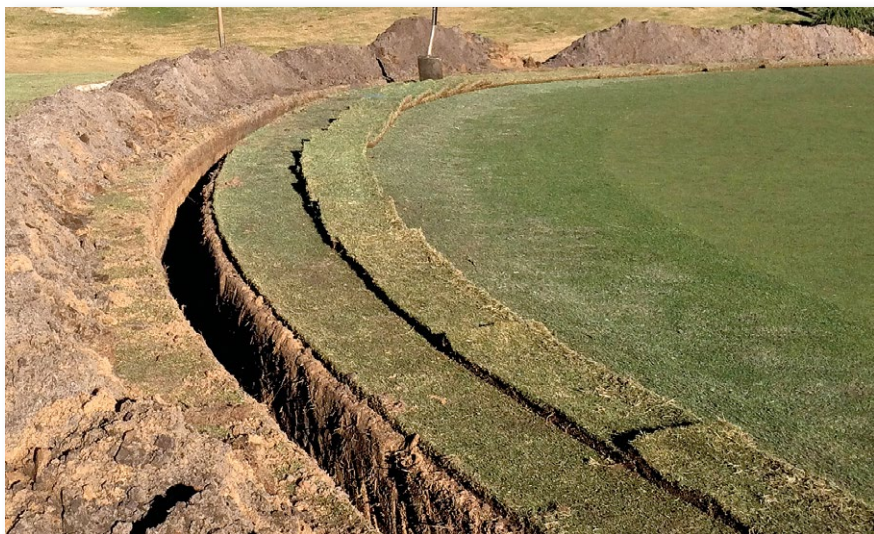
◀ Installation of the 63mm ring main on the 9th green. To minimise disturbance to the edges of greens, the decision was made to dig all greens irrigation trenches by hand. Pictured right is NSWGC crew member Simon Beilby
