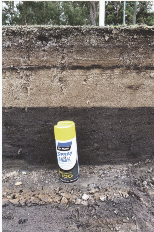
Some interesting profiles were discovered when the old greens were ripped up. The bottom 250mm of this green was virtually impenetrable
