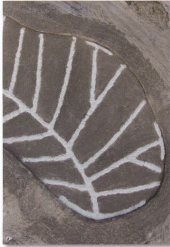
The starting point for drainage design in any sports turf construction should be from the outlet point (lowest point) back to the highest grade point to ensure there is adequate fall available
