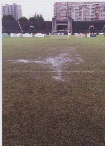
A lot of work was required to get the ground up to AFL standard due to the poor uniformity of the surface
