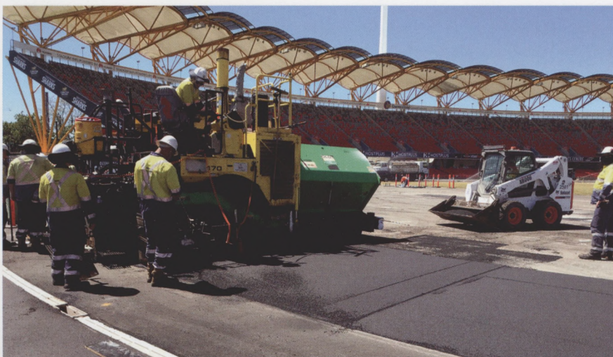
Paving the main competition track within Carrara Stadium
