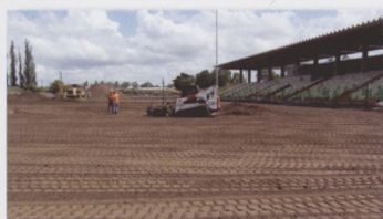
The surface was laser levelled prior to turfing
