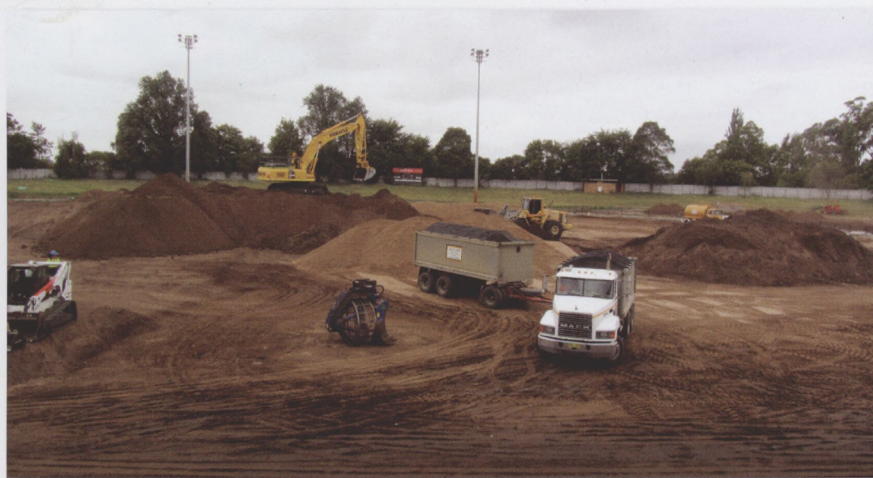
The new rootzone material was blended on site
