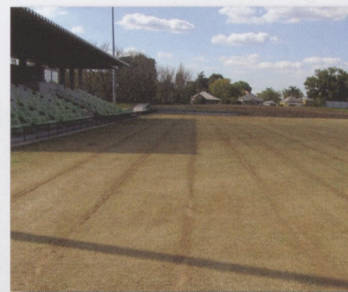
The second stage of the surface redevelopment was the installation of a sand slit drainage system
