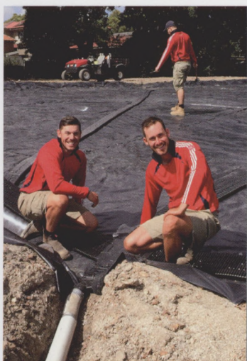
Concord crew members James Strong and Joe Claysey installing drainage on the 17th green. Due to the short timeframe, the bases were covered with a thick plastic to minimise potential of the base being compromised
