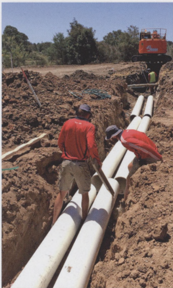
In addition to redeveloping the playing surfaces, Concord also took the opportunity to upgrade its irrigation mainline and install stormwater pipe to direct rainwater from the clubhouse car park to the dam
