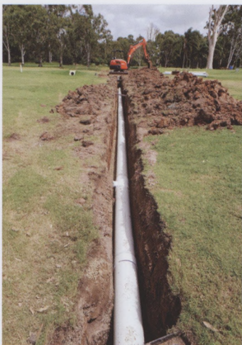
Hervey Bay GC is currently upgrading its fairway drainage infrastructure
