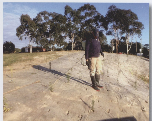
Dominic Bowd spot-sprays weeds that have managed to penetrate the jute matting
