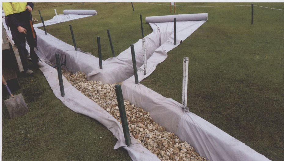
To remedy major drainage issues on lower parts of the course, Watson installed large rubble drains which have proven very successful
