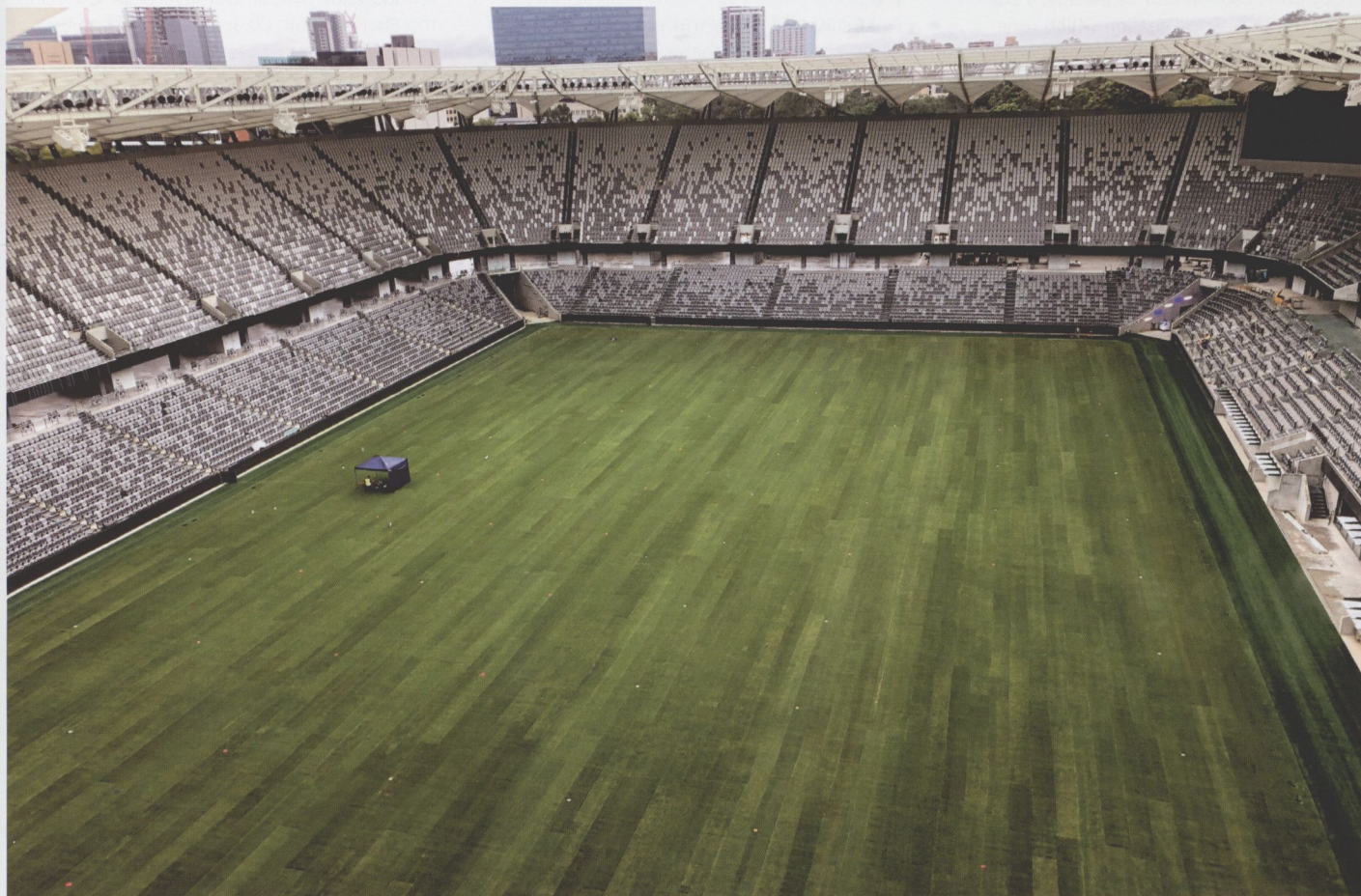
It took HG staff four days to install the 11,400m 2 of Eclipse Stabilised Turf which had been growing at Greenlife Turf in Windsor for more than a year
