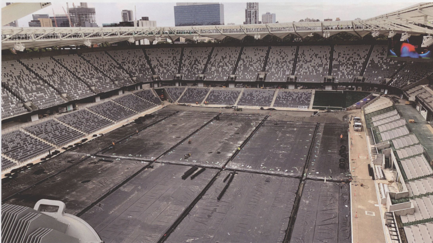
Bankwest Stadium is the first in Australia to use the AirPat vacuum-ventilation system which can force air into the profile and draw moisture out of it. The system comprises a series of feeder and collector pipes on top of a water and air tight rubber liner that covers the entire surface
