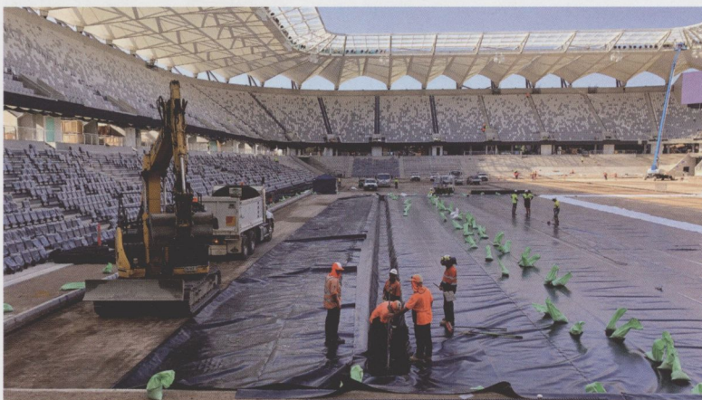
Bankwest Stadium is the first in Australia to use the AirPat vacuum-ventilation system which can force air into the profile and draw moisture out of it. The system comprises a series of feeder and collector pipes on top of a water and air tight rubber liner that covers the entire surface
