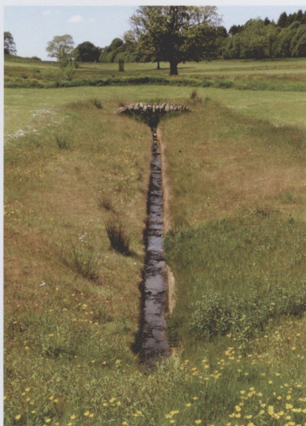
A stone-lined drain, known in Scotland as a 'cundy', was discovered during construction and, with the top stone removed, features on two holes
