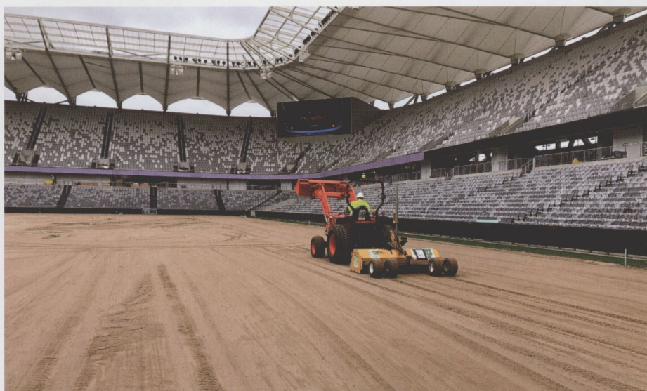
To ensure the surface stayed on grade and within the very fine tolerances set, a Lawless laser grade box worked ahead of turf installation
