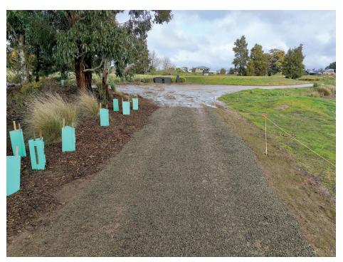
Infiltration rates in field tests on pavement laid by road paver have shown the material to be very effective as a drainage medium.
