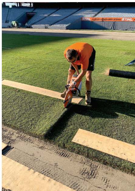
Around 2000m 2 of HERO turf was installed each day with the resurfacing completed in seven days
