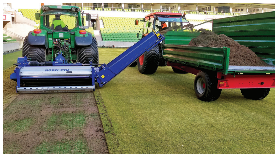
Above: A Koro field topmaker was used to initially strip back the AAMI Park surface to expose the artificial fibres
