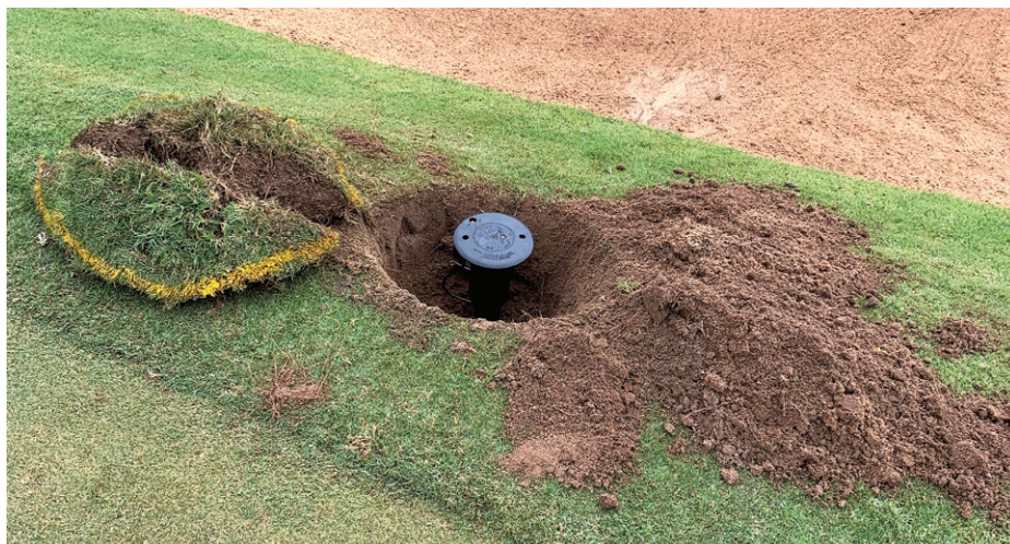
Toro 835 sprinklers are being installed around all Atherton's greens
