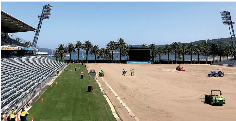
Due to high existing nematode numbers, prior to resurfacing the stadium's profile was fumigated by Melbourne-based Draslovka Services using a product called EDN
