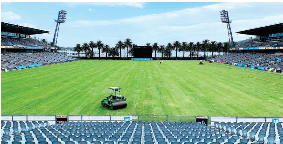
HG's programme allowed for five days to install the new surface, with around 2500m 2 of turf harvested by the crew at the farm each day and freighted the two-hour journey to Gosford
