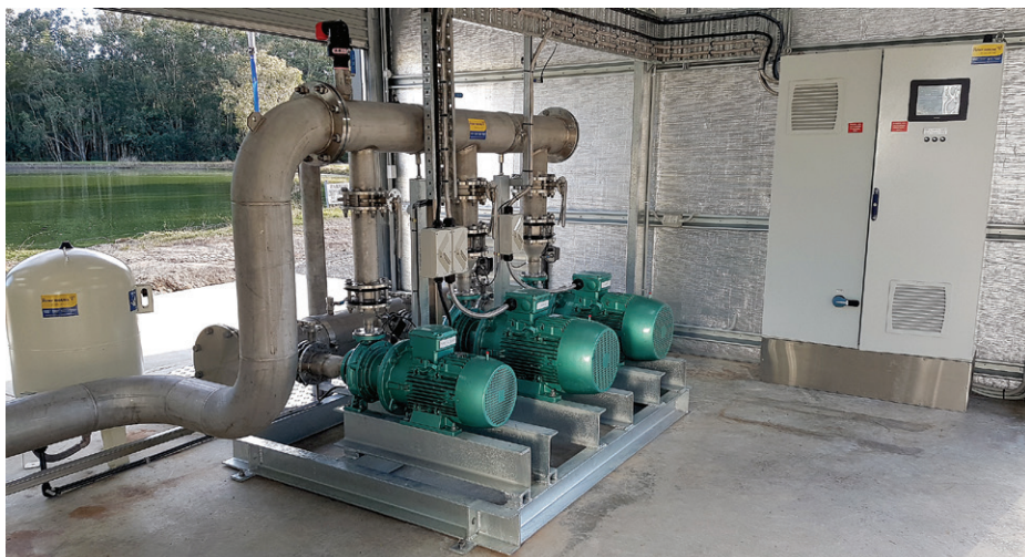
The new multiple pump unit at Twin Waters with variable speed drives in a control panel that has remote device access which is fully interfaced with irrigation central control and advanced flow management system
