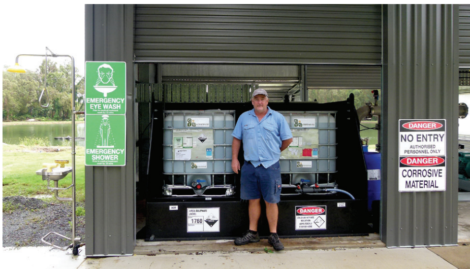
Left: Twin Waters superintendent Garry McClymont in front of the new pump shed showing bunded dosing skid, IBCs (acid, calcium), drum (surfactant), safety eye wash/shower, extra roller door height for IBC access and safety signage
