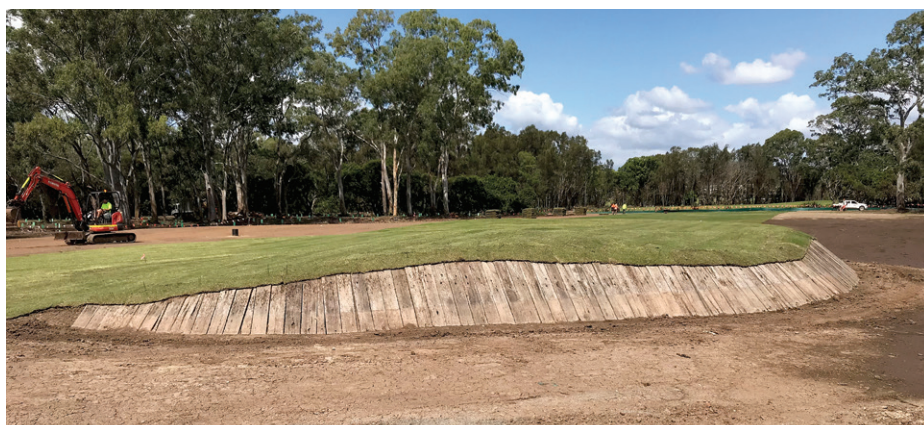
Due to the Minnippi course being located on a floodplain, PCD didn't include any sand bunkers in the design, instead incorporating unique timber faced mounds which will act as hazards
