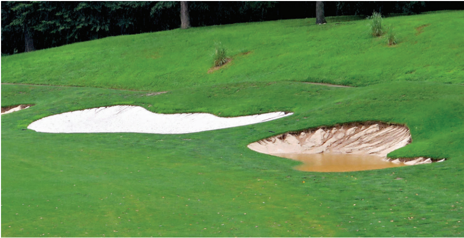
The difference between lined (left bunker) and unlined bunkers is tremendous. Investing in liners yields more reliability and a longer life expectancy for the sand
