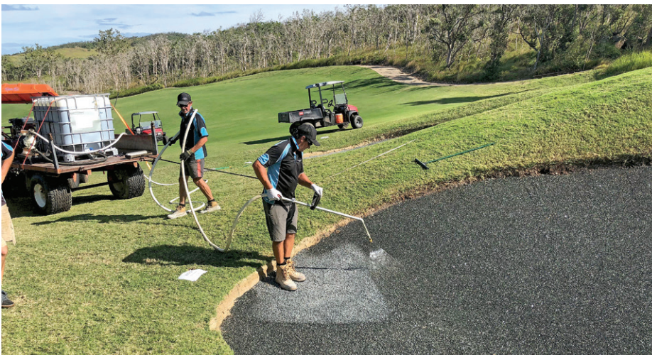
Based on current technology and field experience regarding bunker construction, installing a liner – either a durable liner or a sod liner – is a good idea to keep native soil and rocks from migrating into the sand
