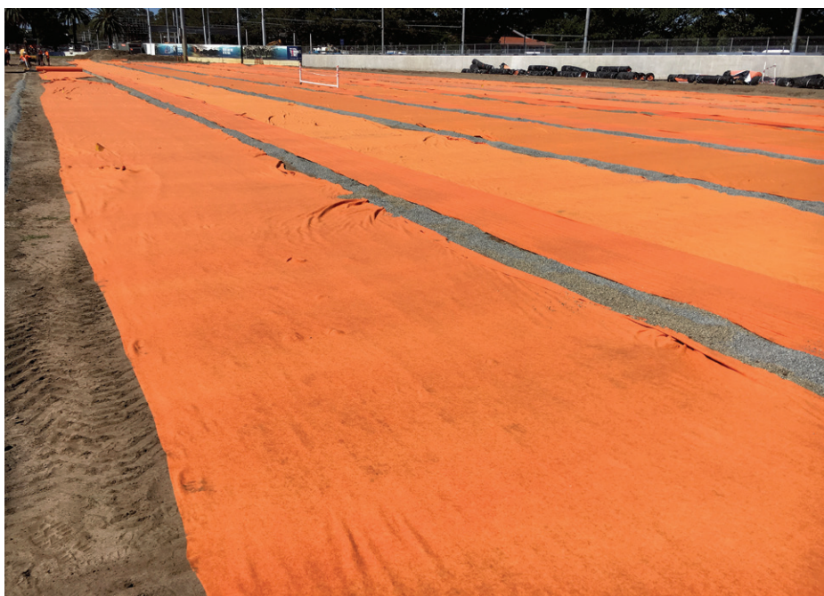
It goes without saying that it's important to know what you are building on. Where contaminated soils are detected, it may be required to lay an orange geofabric as an indicator that there are contaminated soils below
