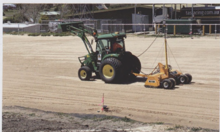
A lower sand layer is laser levelled (left) prior to StrathAyr's reinforced matrix layer being placed
