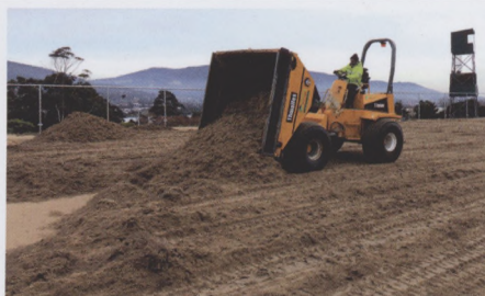
A lower sand layer is laser levelled (left) prior to StrathAyr's reinforced matrix layer being placed
