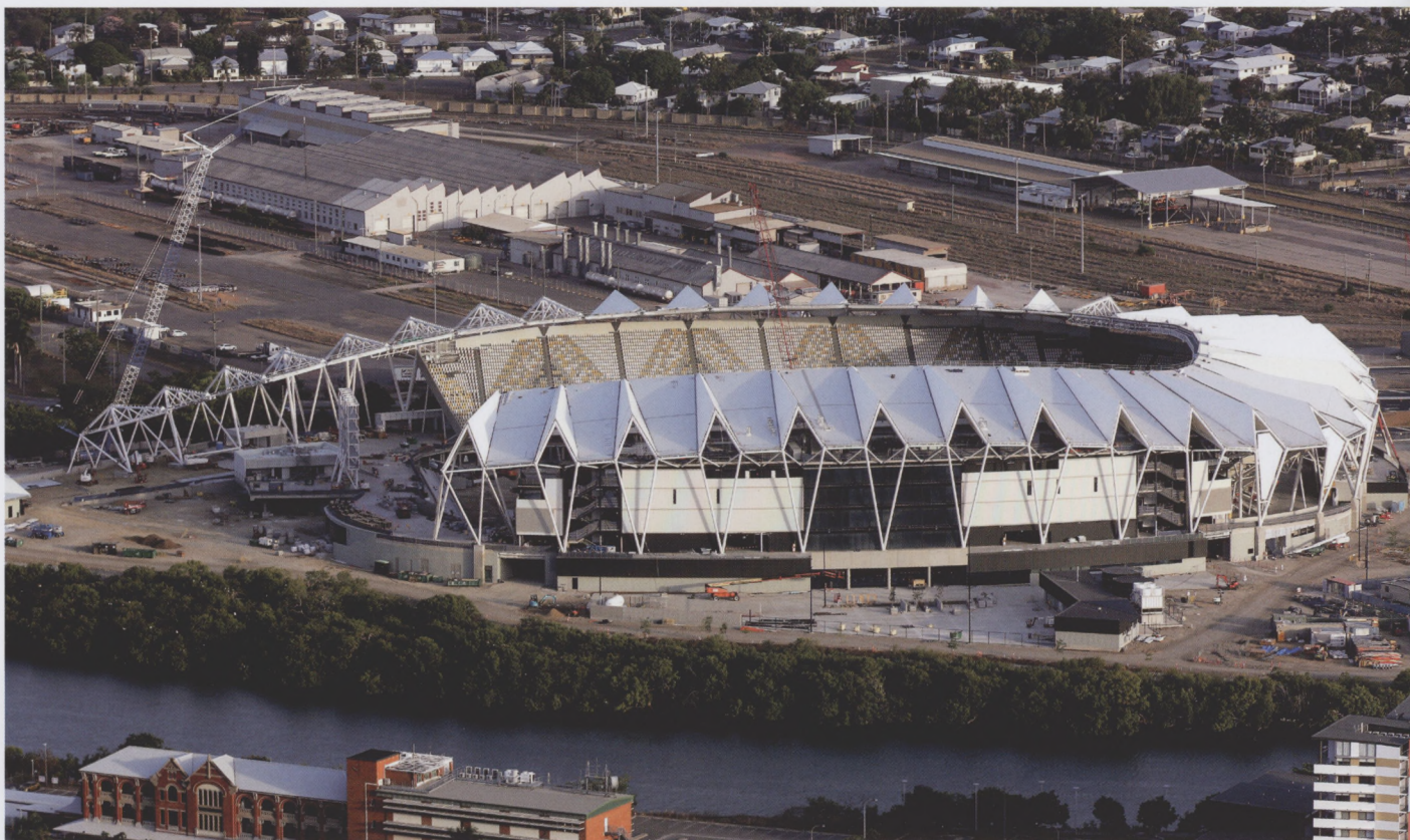
The new 25,000-seat North Queensland Stadium is located in the heart of Townsville and features a horseshoe-shaped, cantilever roof inspired by the pandanus plant
