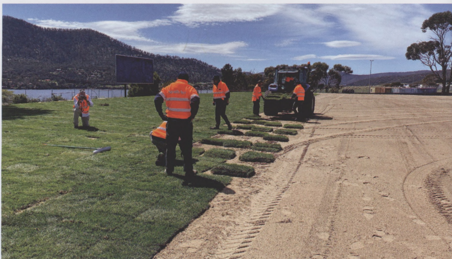
Some 65,000m 2 of Kentucky bluegrass/ryegrass washed turf was used on the new 28-metre-wide Course Proper
