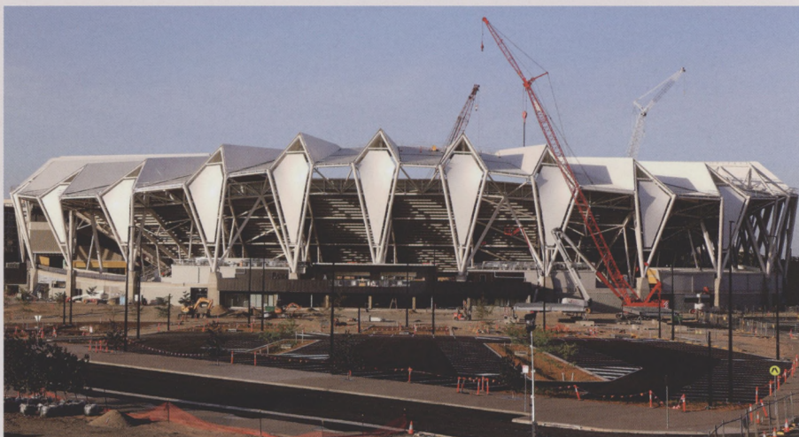
In place of traditional trusses, folded plates achieve the new stadium roof's 'pandanus' geometry. These plates provide strength to resist cyclonic wind loads and flexibility to allow the roof to expand and contract with tropical temperature fluctuations
