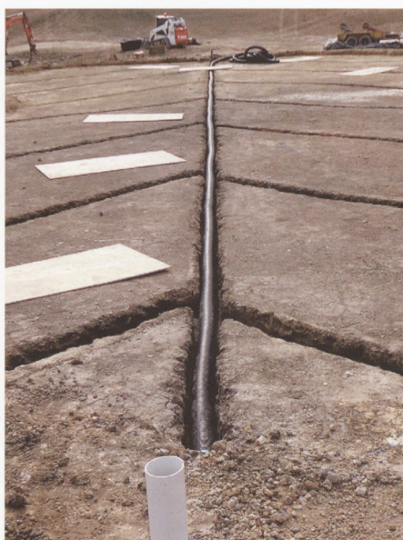
Drainage controls the most fundamental need of a green to grow healthy grass and take traffic without excessive wear or compaction
