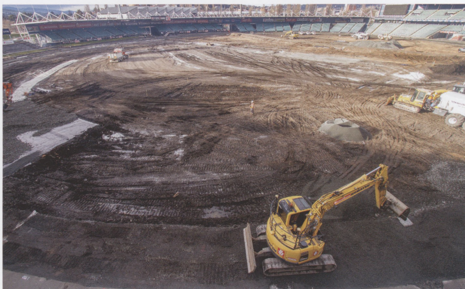
Due to the soft nature of the existing subgrade, stabilising it was a critical component of the project
