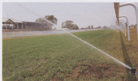
Placement of rotors in relation to the running rail is important to ensure minimal interference with the rotor stream and safety of the horses
