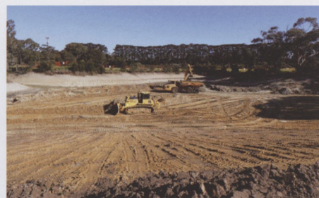
Stage 1 works saw Sandringham's existing irrigation dam expanded from 15ML to 30ML
