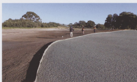
Hydroseeding the fescue surround on 18 after first seeding directly into the soil. A barrier was installed to achieve a hard line between seeding the bentgrass green and fescue surround
