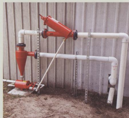
*Sand filters are attached to each pump*
