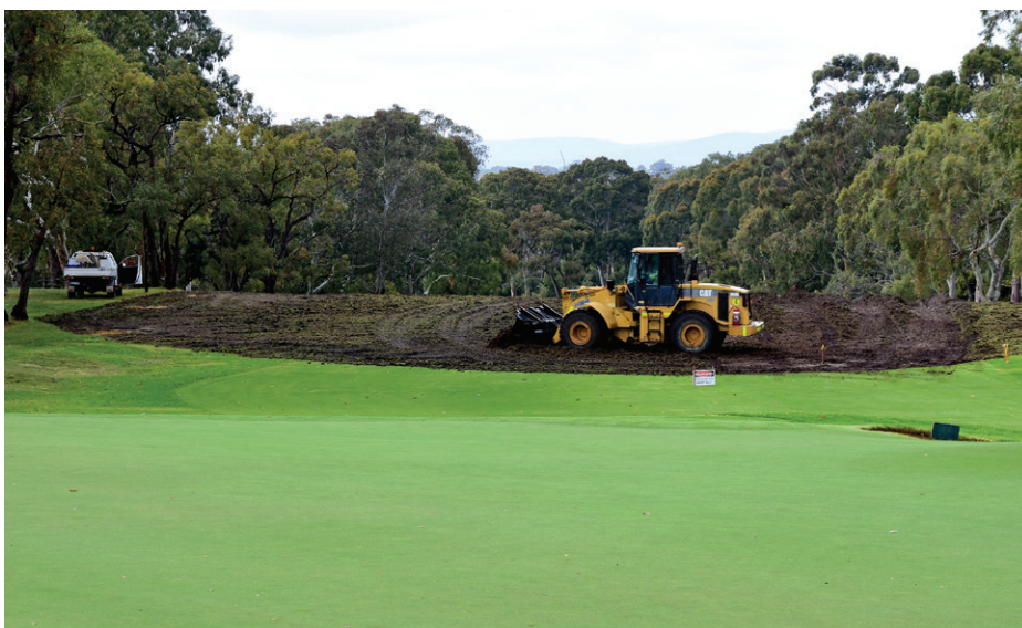
Grubbing the ridge in front of the 18th green. The ridge, about 100m-120m from the green, meant a second shot into the green was blind. Removing it has helped to improve playability and aesthetics
