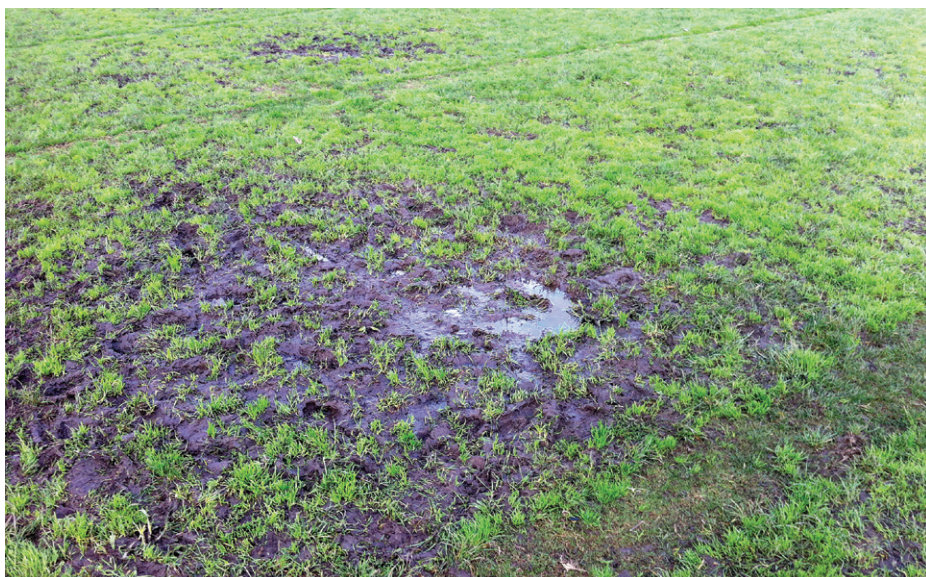
Sports fields constructed with wider drain spacings, often in order to save money, will ultimately provide an inadequate playing surface due to the drainage system's inability to remove water quickly and effectively
