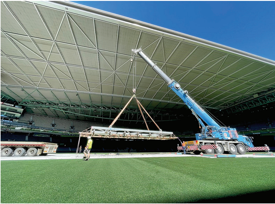
Marvel Stadium has four drop-in wickets – two for the centre and two for the practice areas. Each pitch is transported in two sections by truck and carefully lowered into position. The whole process takes a full day
