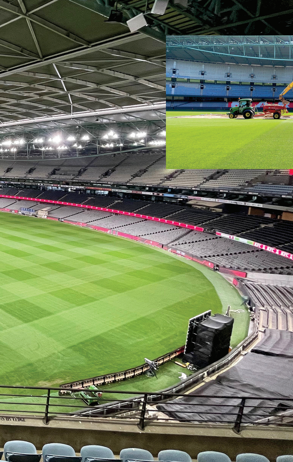
Above: The drop-in process requires 650m 2 of turf and 50m 3 of sand to be excavated and graded to the required level
