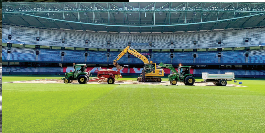
Above: The drop-in process requires 650m 2 of turf and 50m 3 of sand to be excavated and graded to the required level
