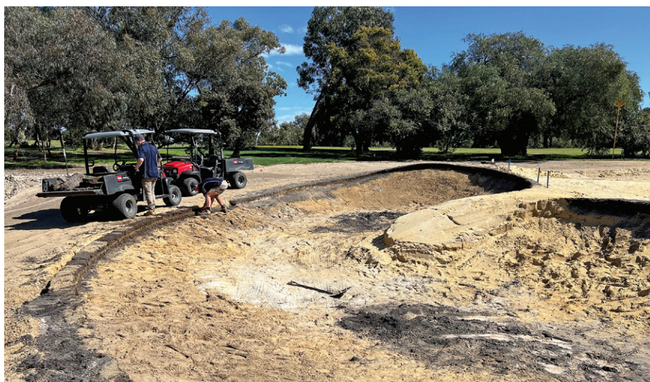
100mm-deep Santa Ana sod has been used torevet the new bunker edges and provide a lip on the short grass side
