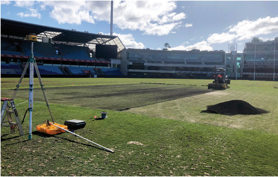
As part of the wicket table renovation, the AFL centre circle area was milled out to remove any trace of paint pigment. Fresh wicket soil was then incorporated and laser levelled before being reseeded
