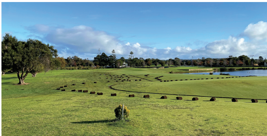
Above: About 1600 lineal metres of herringbone drainage has been installed on the Dunsborough Lakes fairways in recent years. Pictured is the 18th hole. Right: All couch surfaces are aggressively scarified each spring
