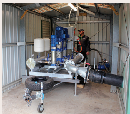
Beenleigh RSL and Golf Club's irrigation pump station was recently upgraded with a custom-made mobile booster set that can be transported to higher ground in the event of flooding
