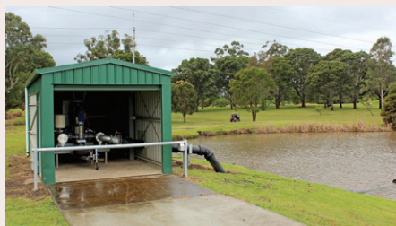
Beenleigh RSL and Golf Club's irrigation pump station was recently upgraded with a custom-made mobile booster set that can be transported to higher ground in the event of flooding
