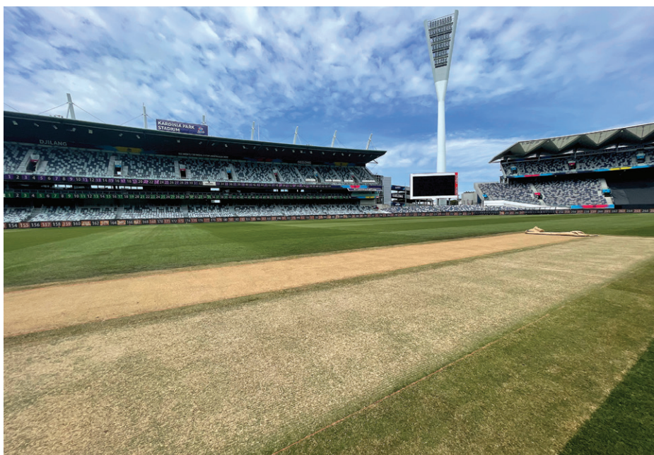
Kardinia Park's older drop-in wicket (foreground) is more than 10 years old and constructed with Gabba wicket soil from Queensland. The newer wicket constructed in 2019 was built with clay sourced out of Dunkeld in Victoria's Western Districts
